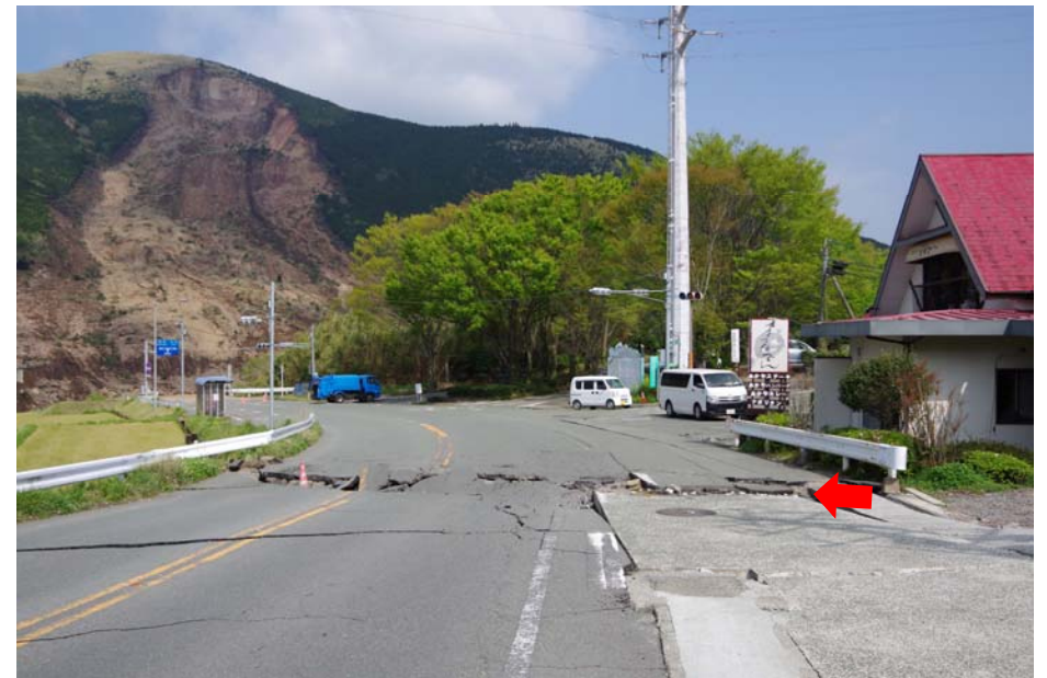
Ruptures running toward the village
