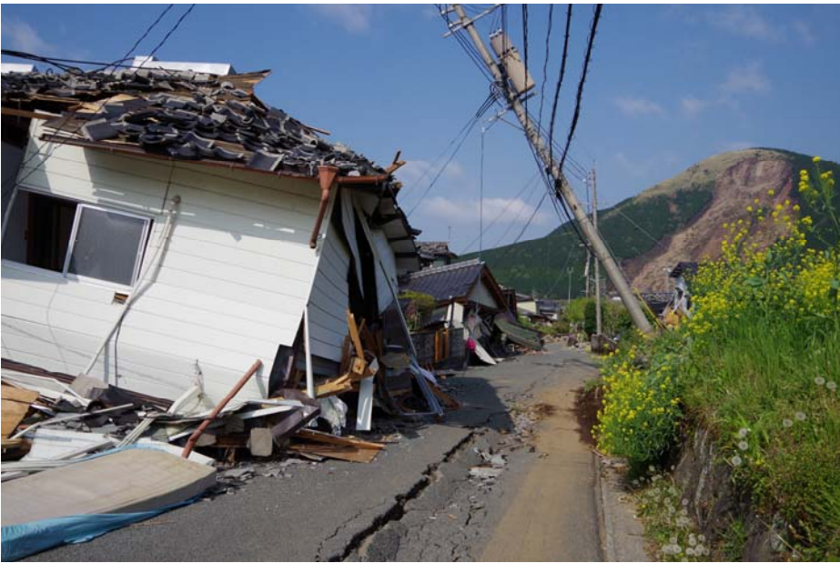
Collapsed Houses in the vicinity of the earthquake fault
