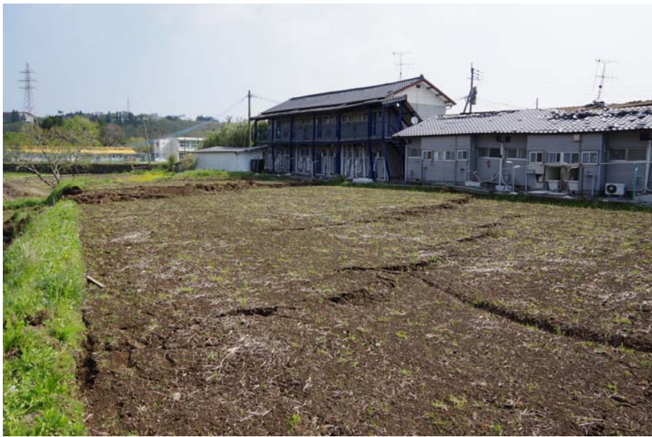
Houses just on the earthquake faults
