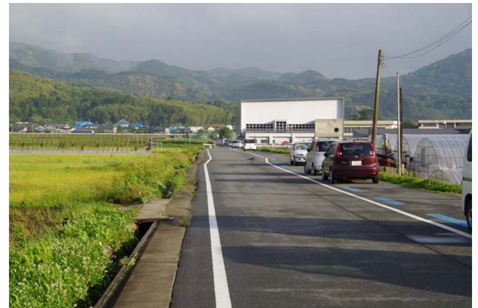
Branching fault in the Mashiki town
