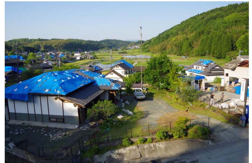
Branching fault in the Mashiki town
